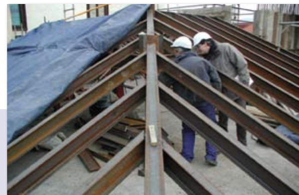
New roof construction
