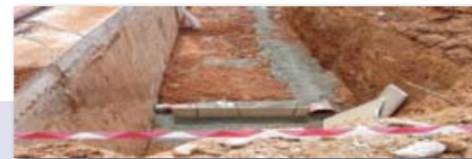
Ground heat exchangers for cooling
