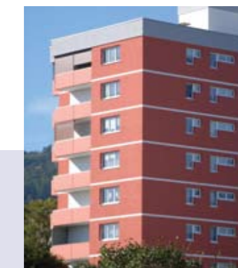
After the renovation
