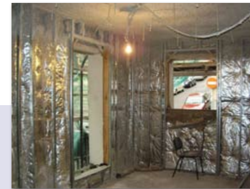
Internal insulation with vapour barrier
