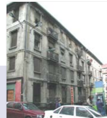
Before the renovation
