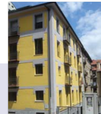
After the renovation
