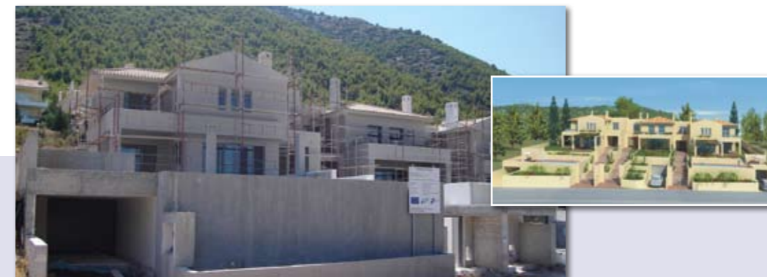
Building 4 onder construction
