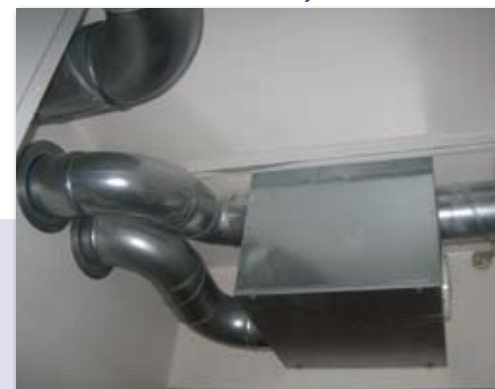
Newly developed heat recovery unit
