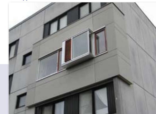
Test apartment after renovation
