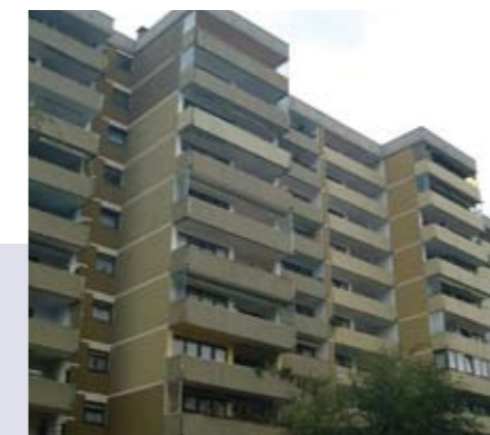
Before the renovation
