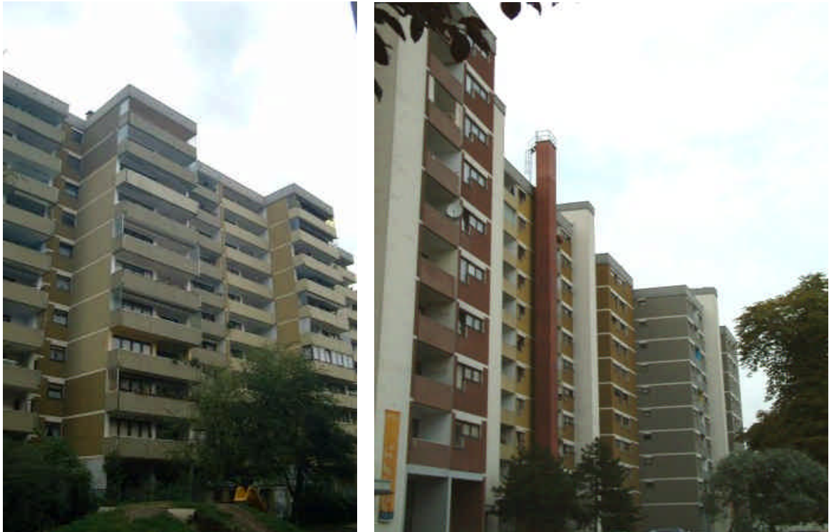
Figure 2. Austria, East and West view of the pilot building
