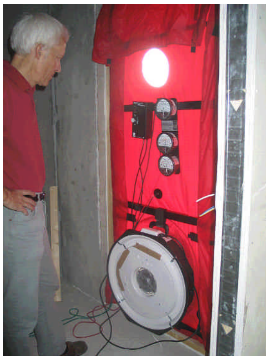
Fig. 8.2.1.: Blower Door test in an apartment.
