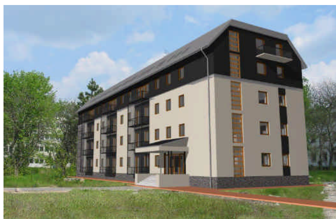
Figure: The project building before and after the retrofit
