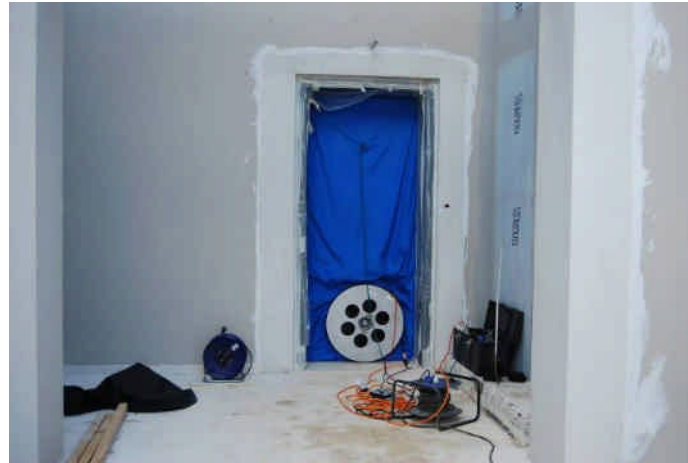
Figure 4.3.1.: Blower door test - entrance of dwelling I2
