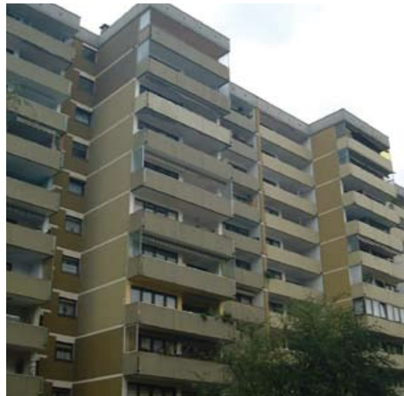
Situation before renovation - West façade
