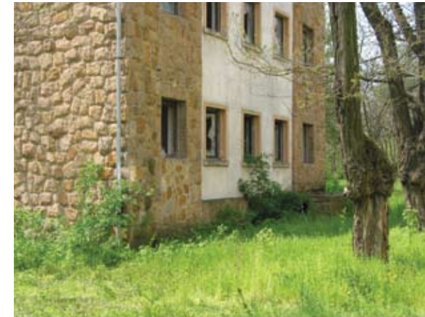
The project building in its recent state
