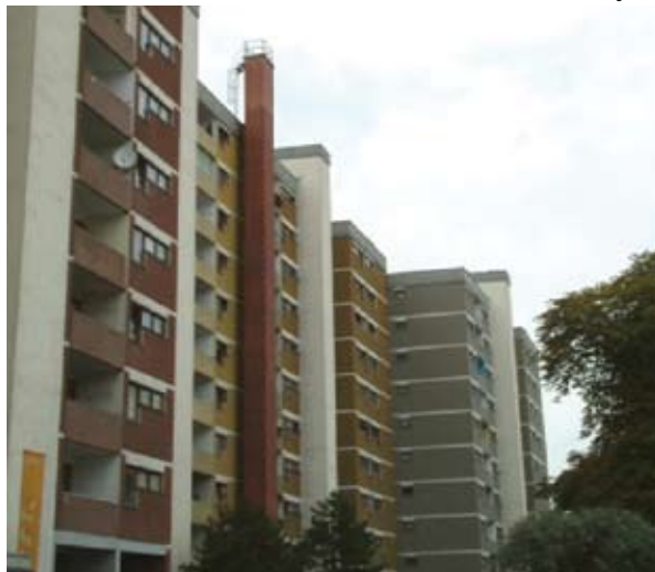
Situation before renovation - East façade
