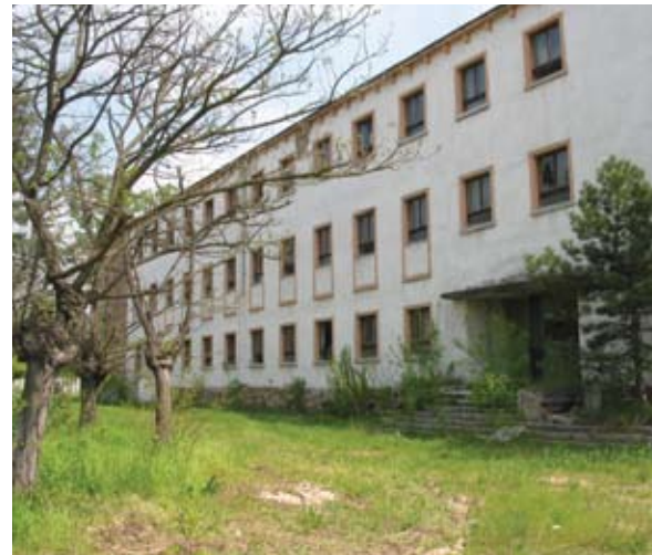
The project building in its recent state
